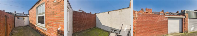
Rear courtyard with a garage accessed via electric roller shutter.
